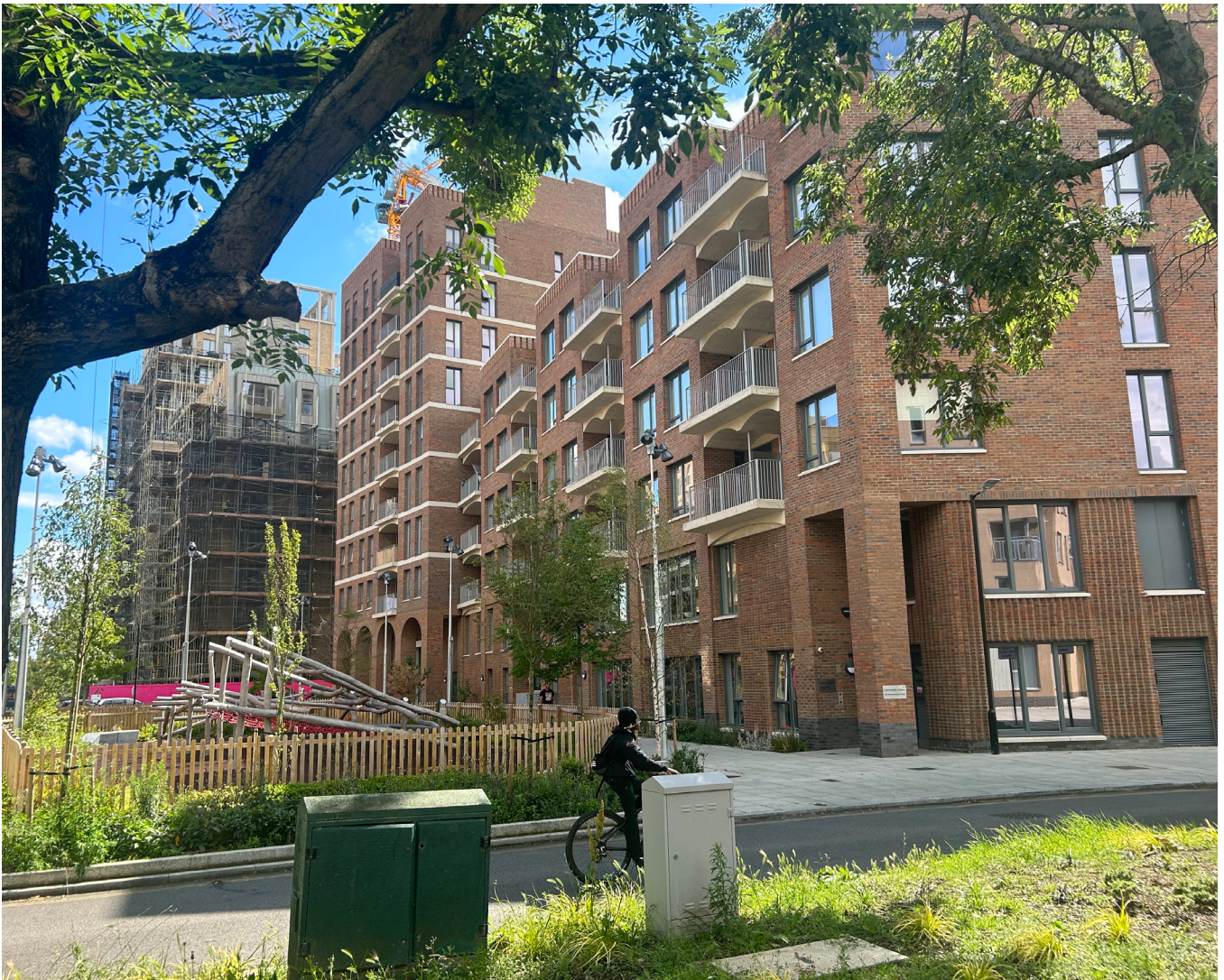
Figure 3: View of completed Phase 1a from Westmoreland Road
