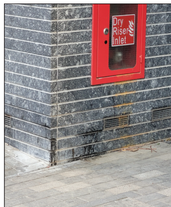
20. Weep holes and vent
