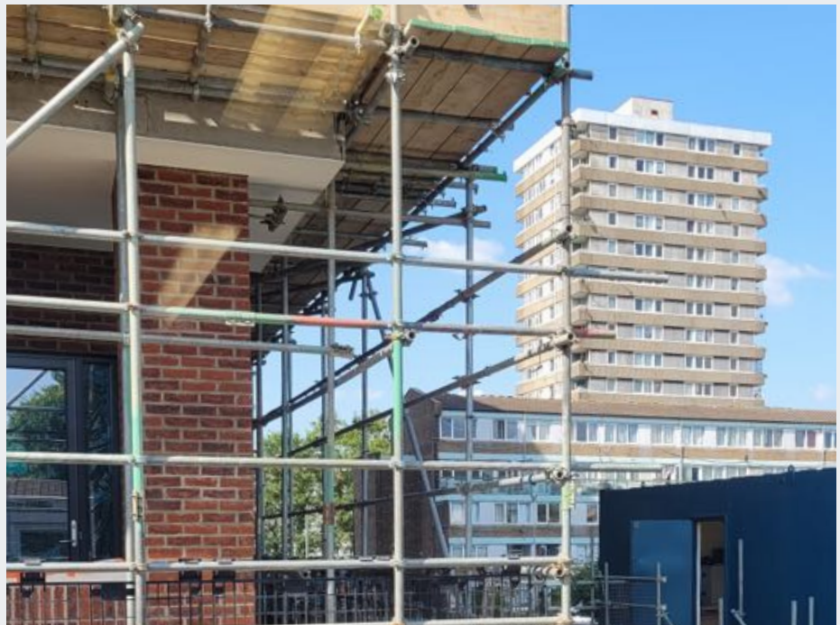
Figure 5: Delivery of Phase 1 Blocks with tower in background
